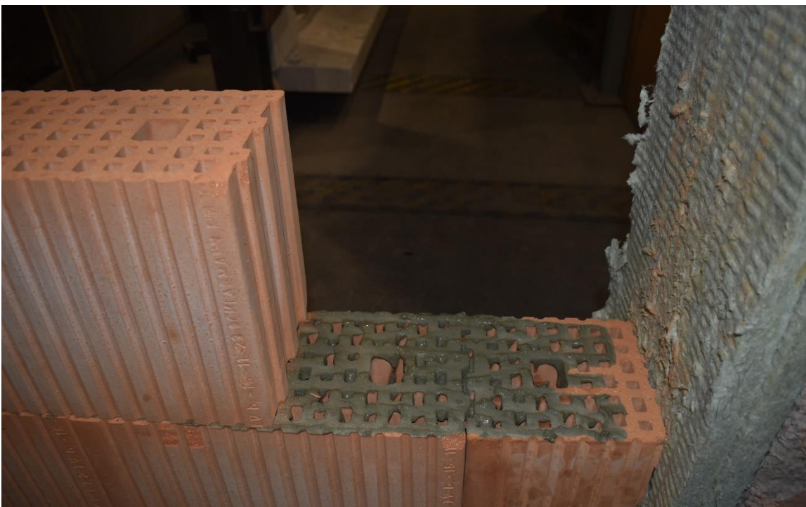
Photo No. 4 Mortar on top of the blocks for placing the next layer of blocks.
