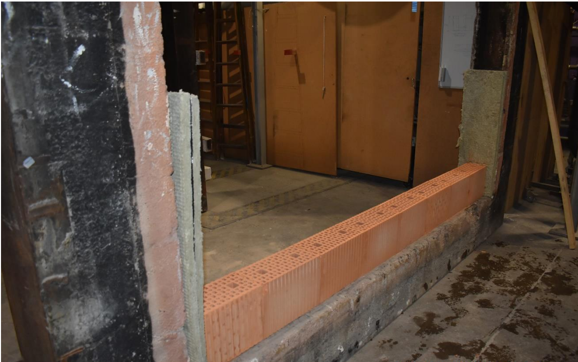
Photo No. 1 Mounting of the first layer in the bottom of the wall.
