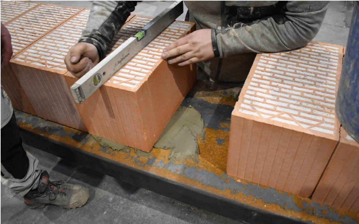
Photo No. 3 The blocks were aligned before placing the next layer
