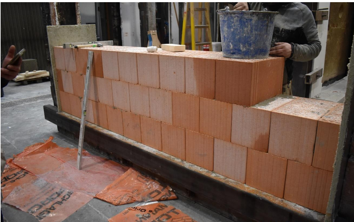
Photo No. 4 Three layers was placed with mortar on top of them
